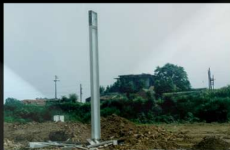
18-3-1997 Piling The First Pillar Of The Engine Factory
